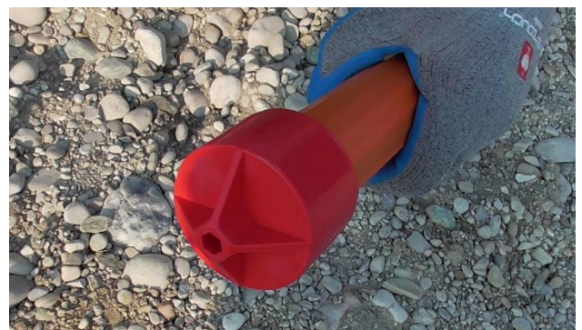
1.7 Final installed sealing cap.
