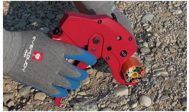
1.3 Cut end of microduct bundle vertical and straight.
