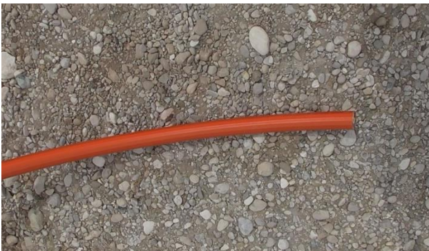
1.1 A temporary sealing cap should be used during transport or installation for microduct bundles. For installation stretch about 1m of duct bundle.
