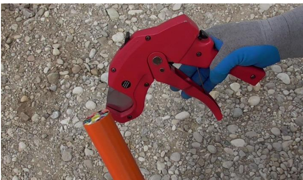
1.2 For cutting end of microduct bundle use a tool recommended by duct manufacture.
