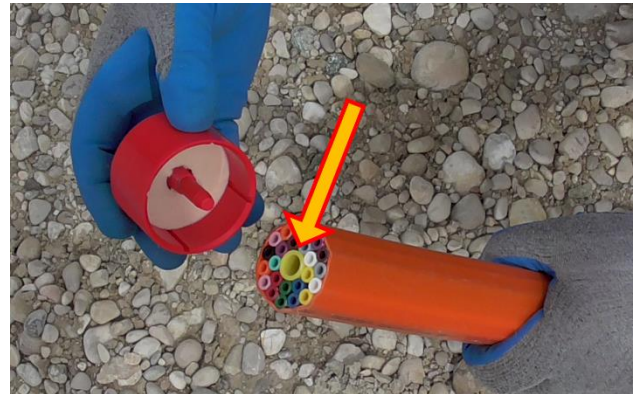
1.5 Position central thorn in front of central tube from microduct bundle.
