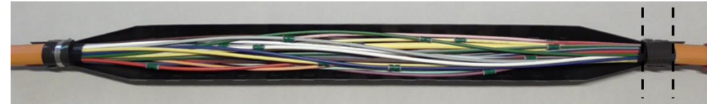
1.15 After all microducts have been connected, still loose side of microduct bundle need to be fixed. Install rubber stripe and duct bundle strain release as described under chapter 1.6 and following. Before fixing of hose clamp, check again if rubber stripe and clamp shell are in right position. Right position is mandatory for full strength of strain relief. Afterwards tighten hose clamp like described under chapter 1.9.
